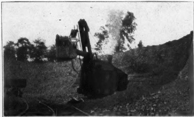
Steam Shovel in Operation at Bank Above Water Line
